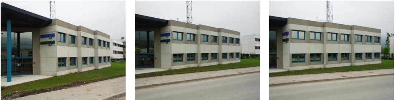
Figure 13: Three out of the six images of the BUILDING dataset. Note the significant parallax of windows relative to the wall.
